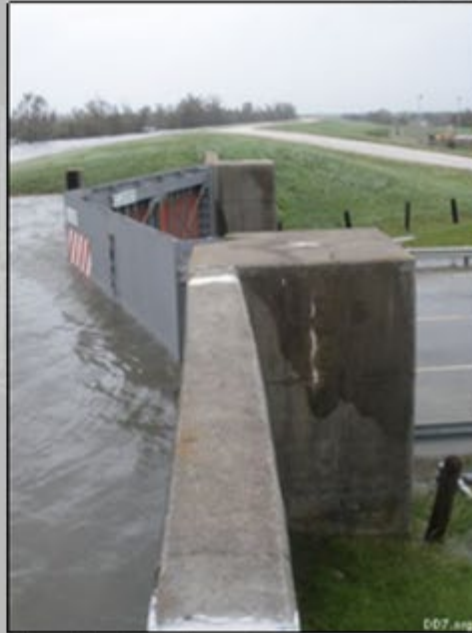
Road closure gate
